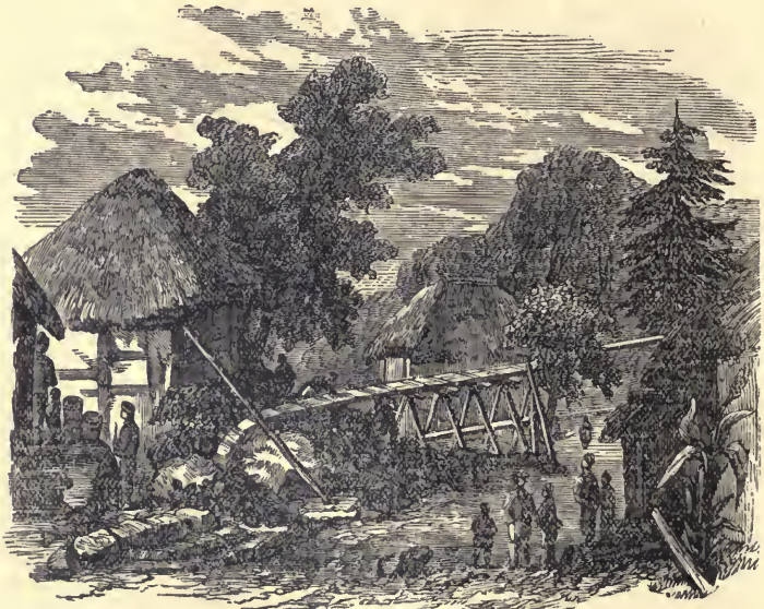
THE VILLAGE AQUEDUCT.
